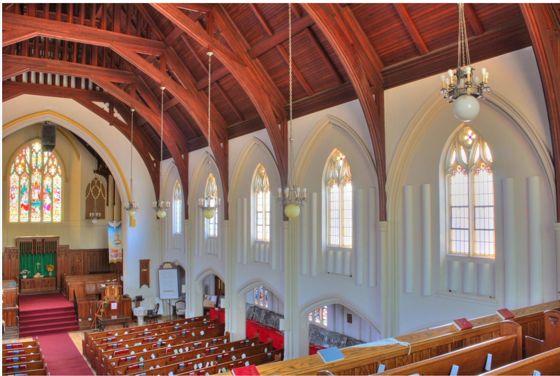
Each section of the side wall targets different frequencies and amount of sound diffusion.
